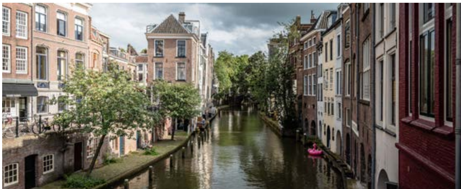
In Utrecht, thousands of houses have inadequate foundations.
