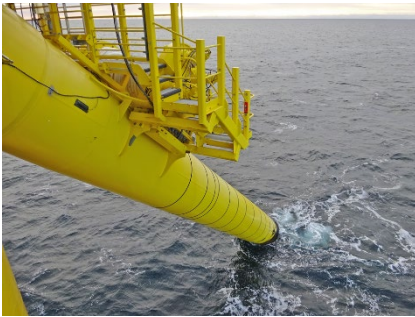
Structural load measurements
