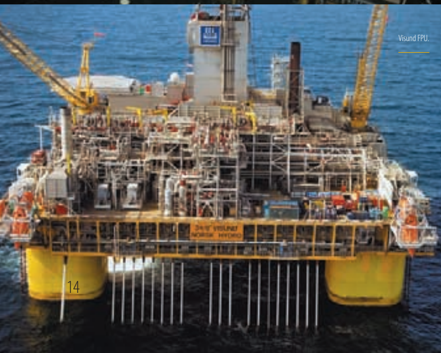
Installation of 2nd module.
