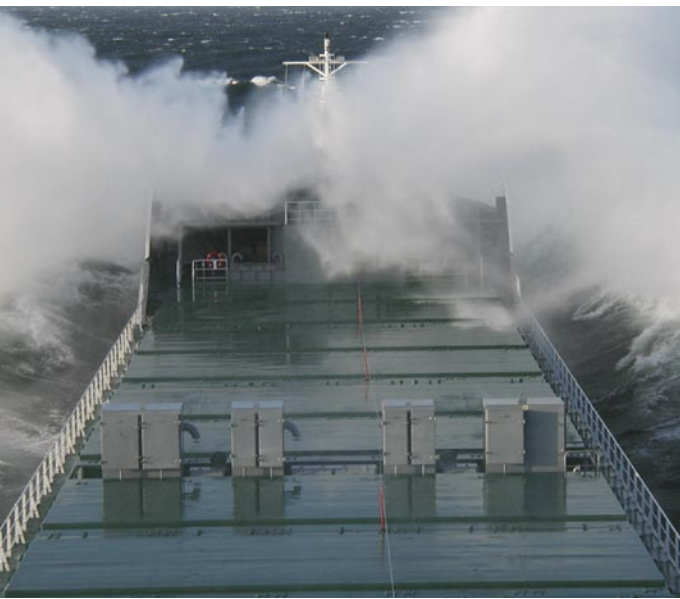
Monitoring impacts and hull strains on Victoriaborg.
