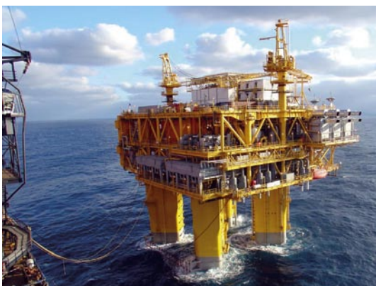
Monitoring motions and loads on Marco Polo TLP in the Gulf of Mexico.
