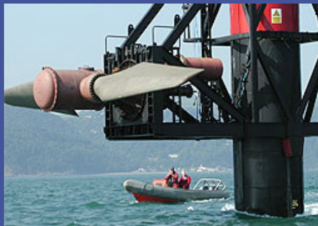
The SeaFlow proof of concept tidal turbine, which has been installed near Lynmouth in the UK, since May 2003
